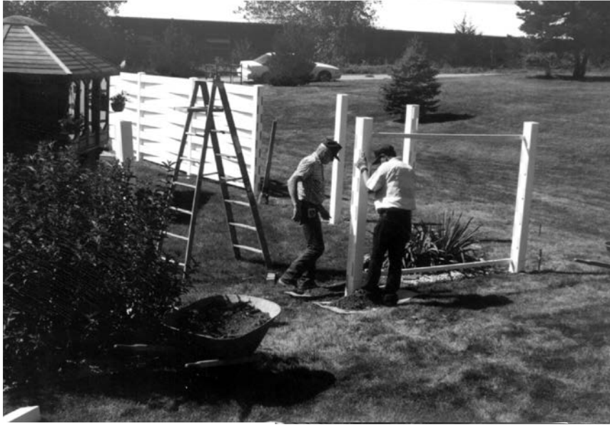
Posts are set for the entire installation.
