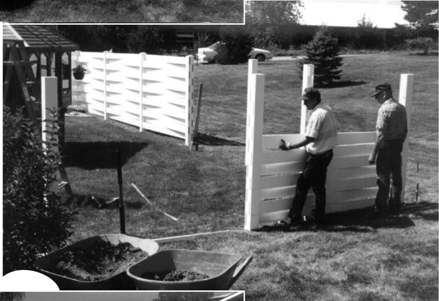
Prebuilt fence sections or horizontals are then mounted to or through the routed posts.
